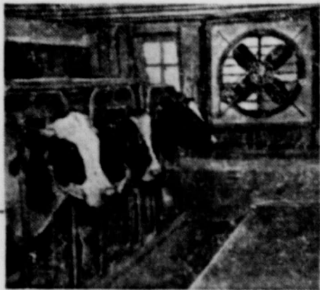
Picture on Vernon Julins farm at Freeport, Ill., shows installation of automatic cooling unit in dairy barn.
