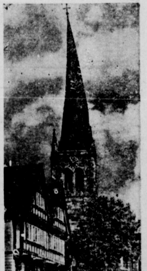
CROOKED SPIRE . . . The famous crooked spire of the parish church, Chesterfield, England. The spire is twisted owing to the warping of the timbers beneath a leaden covering. It is 230 feet high, 8 feet out of perpendicular.
