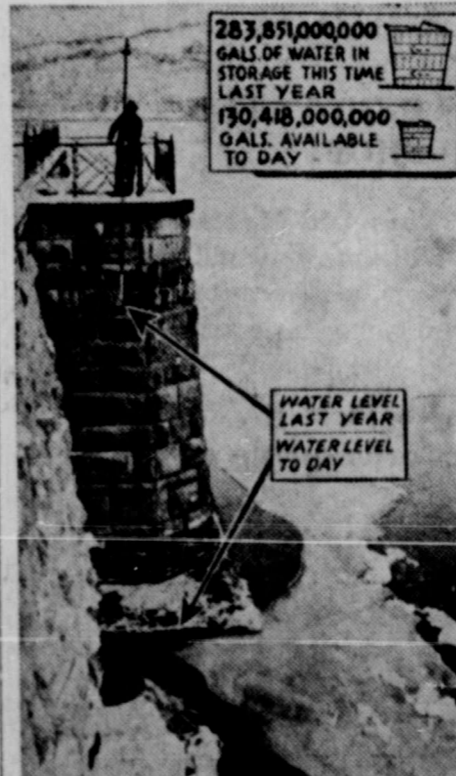
Photo-diagram shows the seriousness of New York city's water shortage, due to last year's drought. The reserve water is only 46 per cent of the 1939 total at Croton reservoir. Gatehouse Foreman John Tompkins indicates with a pole the point to which water usually reaches.
