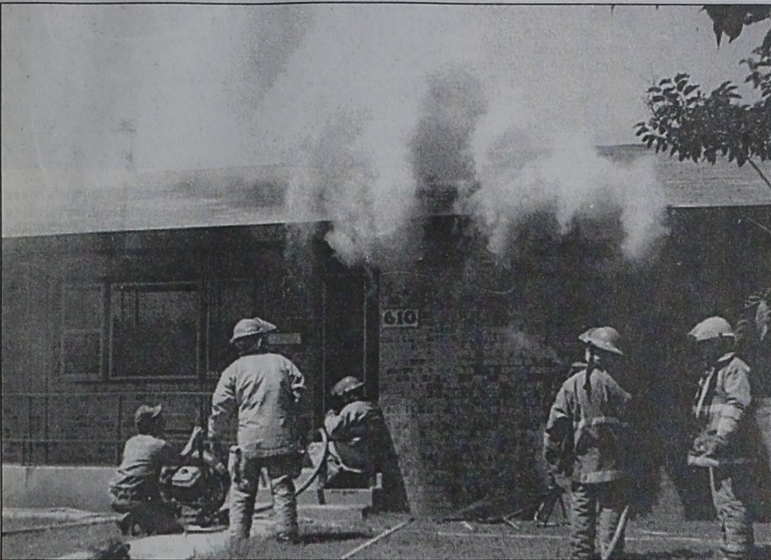
HEAVY DAMAGE to one bedroom and extensive smoke and heat damage throughout the house resulted from this fire at the home of Monticello Flores at 610 W. Stinson in Dimmitt last Thursday at 3:10 p.m. Fire Chief Tommy Cleavinger said it is
