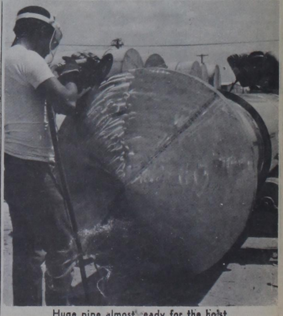
Huge pipe almost ready for the hoist
