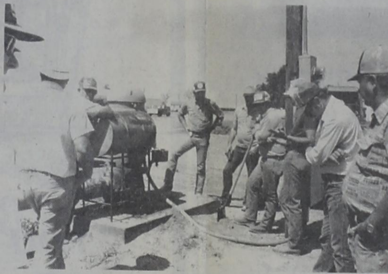
Shown is Jerry Funk, with the High Plains Underground Water District, explaining the procedure for running a well evaluation on an electric motor, to a group of producers attending our annual irrigation field day.
