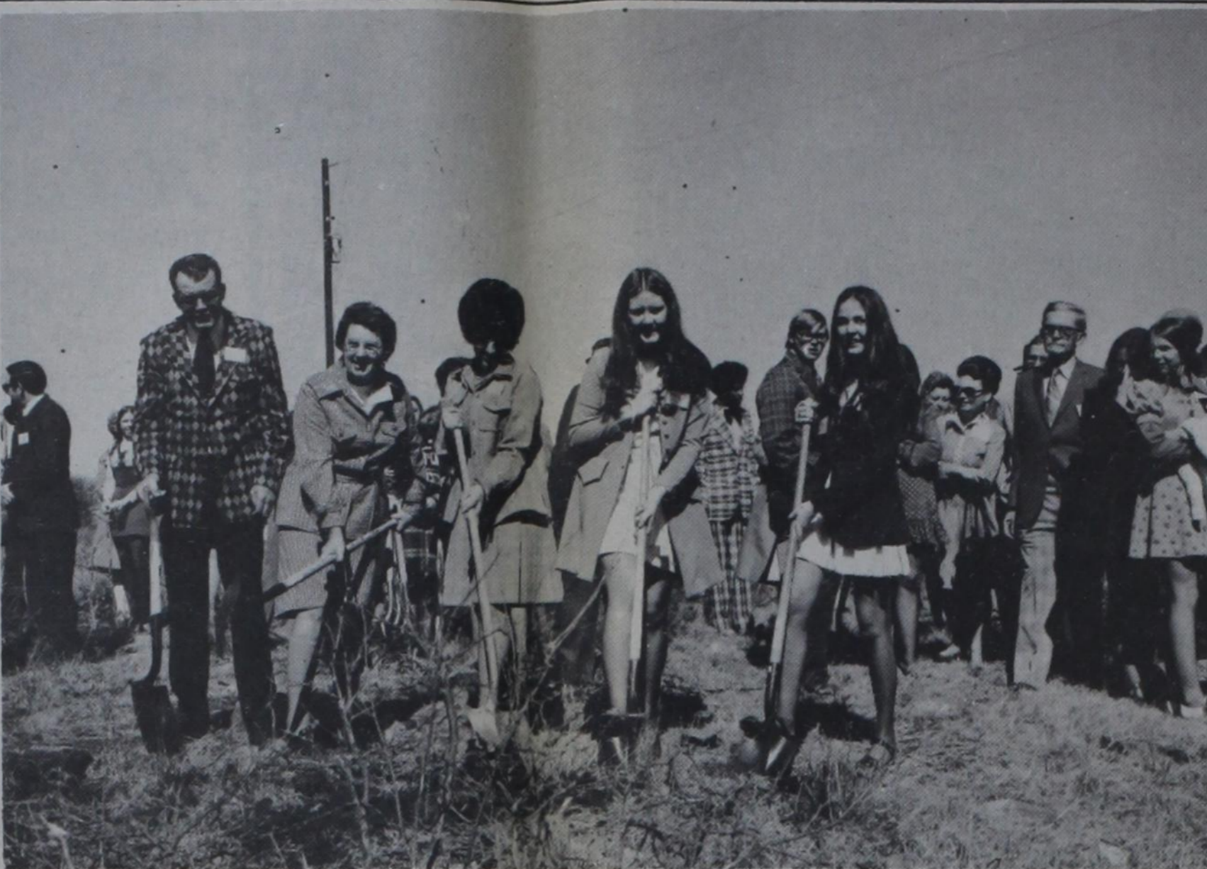
CONSTRUCTION on Texas' new $1.375 million 4-H Center got underway on a scenic 78 acre site overlooking Lake Brownwood last spring. Present at the groundbreaking ceremony at the lake site was this delegation from Extension Service District I. Pictured from left to right are Mr. and Mrs. Jack Ingram of
