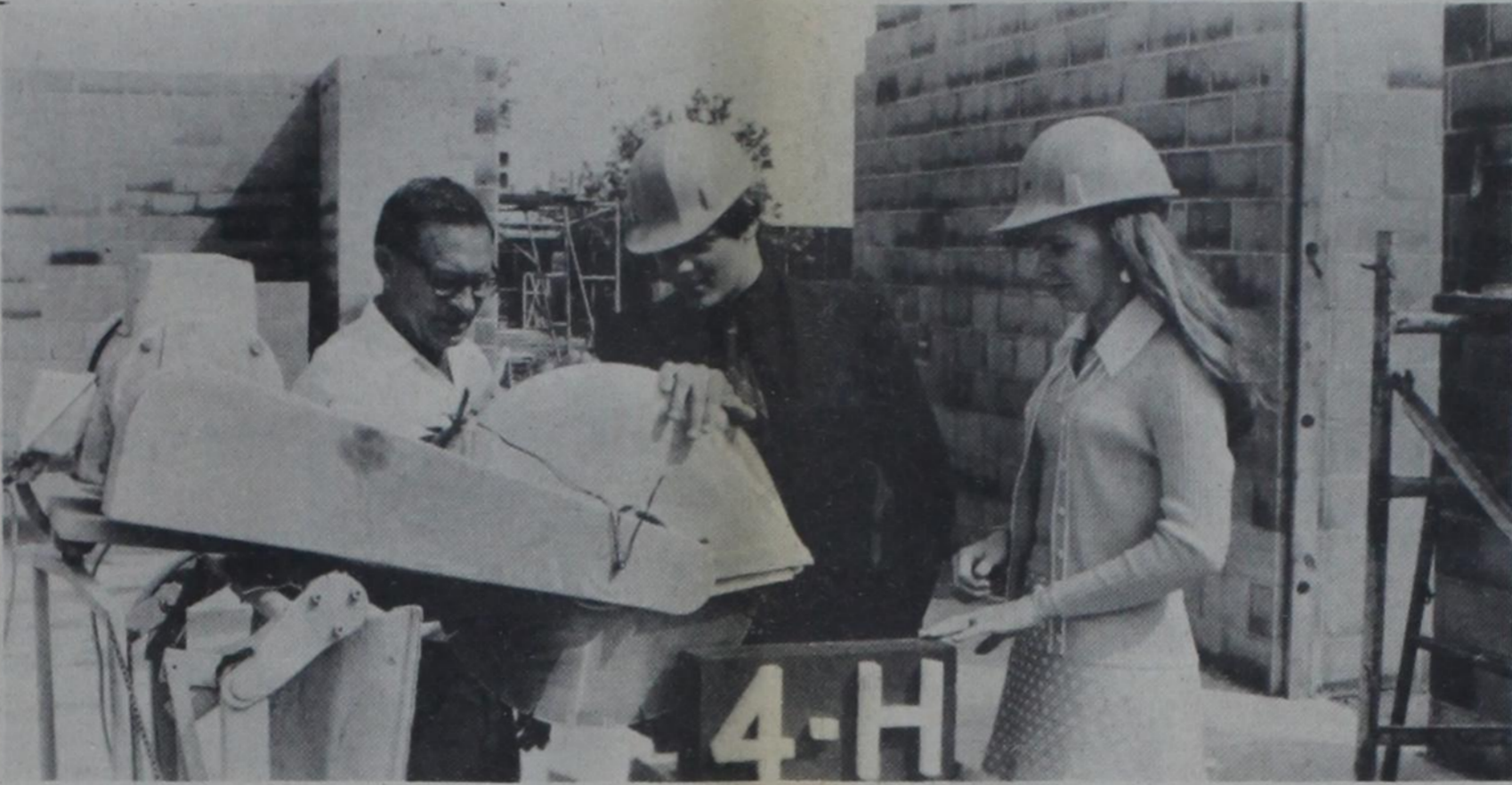
EDDIE PERKINS of Cleburne [center] and Jamie Hemphill of Coleman, chairman and vice-chairman, respectively, of the Texas 4-H Council, inspect a masonry saw with Job Superintendent Ed Miller of the Herman Bennett Company while on a special inspection tour of the $1.375 million Texas 4-H Center at Lake Brownwood. The 200-capacity facility is being constructed under the leadership of the Texas 4-H
