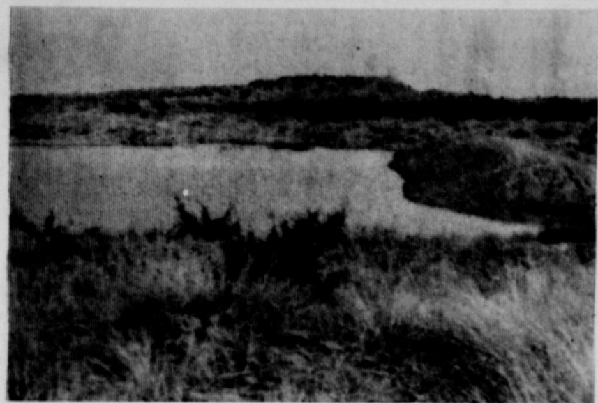
PLENTY OF STOCK WATER —This dam-type pond on the Cumble Ivey ranch southeast of Robert Lee has a storage capacity of 7.76 acre feet, a
