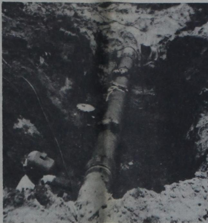
REPAIRING THE BREAK —Working in oil-blackened ground, welders replace the broken section of the Phillips pipeline on the Harold Bob Bennett farm Friday. Spurred by a heavy rain during the night, oil drained across 10 acres of cotton, killing the soil for at least four years. Complaints about the strong odor of the crude oil came from as far away as Hereford.
