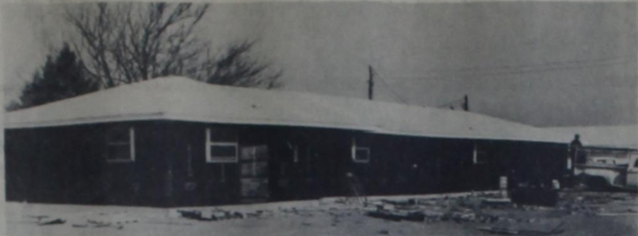
A NEW PARSONAGE is rising from the ashes of the tragic fire that destroyed the Frio Baptist Church parsonage Jan. 12. The new parsonage will be much larger than the one that burned.
