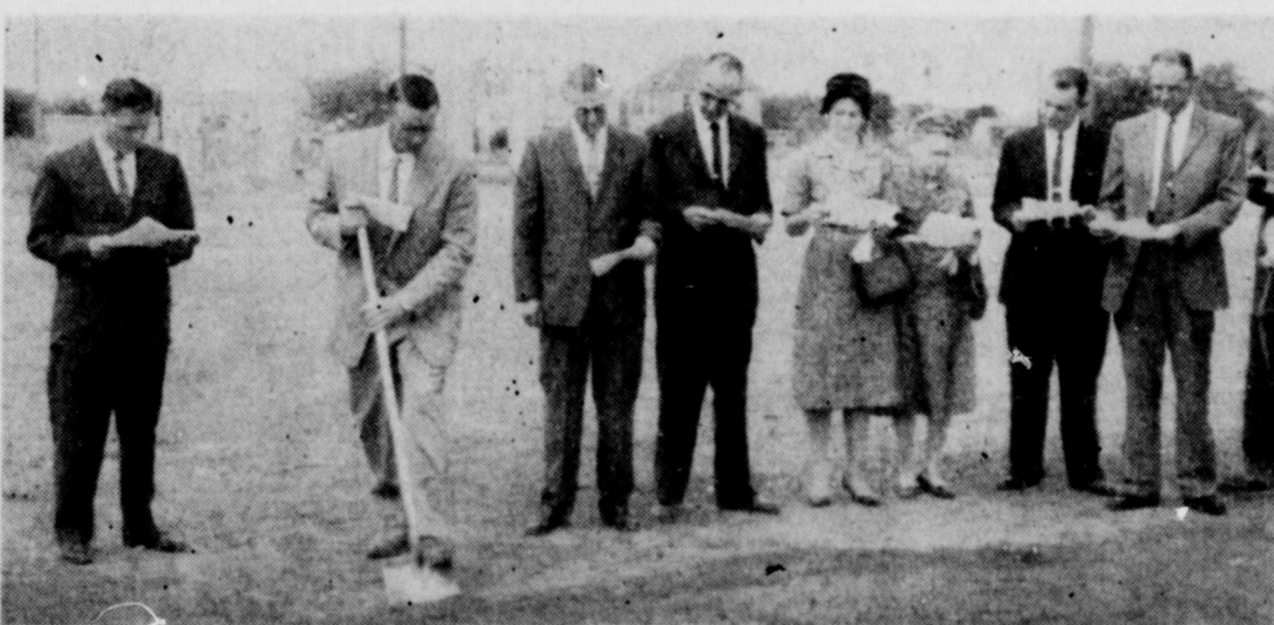
BREAKING GROUND —Conda Richards, chairman of the board of stewards, at First Methodist Church, turns the first shovel
