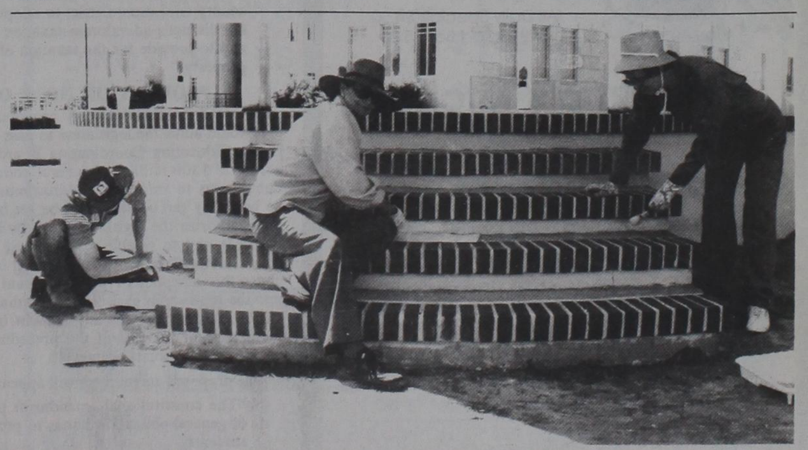
ANOTHER STEP—Dorothy Sheffy (seated) and Myrtle Lois Moran apply colored sealcoat to the steps of the gazebo in the Centennial Plaza Saturday, while Rex Wooten (left) lends a hand to bring the project another step closer to completion. Volunteers also sealcoated the stem-bases of the
