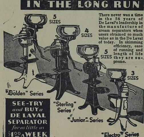
THERE are four complete lines of De Laval Separators, which include 17 different styles and sizes of machines ranging in separating capacities from 150 to 1575 pounds per hour-previding a De Laval for every need and purse. See them.
