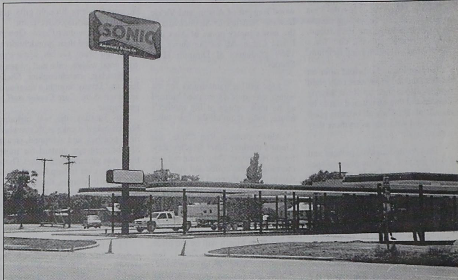
THE SIGN IS UP and work is almost complete at the new Sonic Drive-In, located on the corner of Halsell Street and North Broadway in
