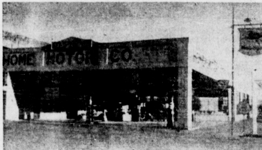
The Home Motor Co., of which Robert Knierim is owner, is modern in every respect. This building also serves as bus and truck depot.
