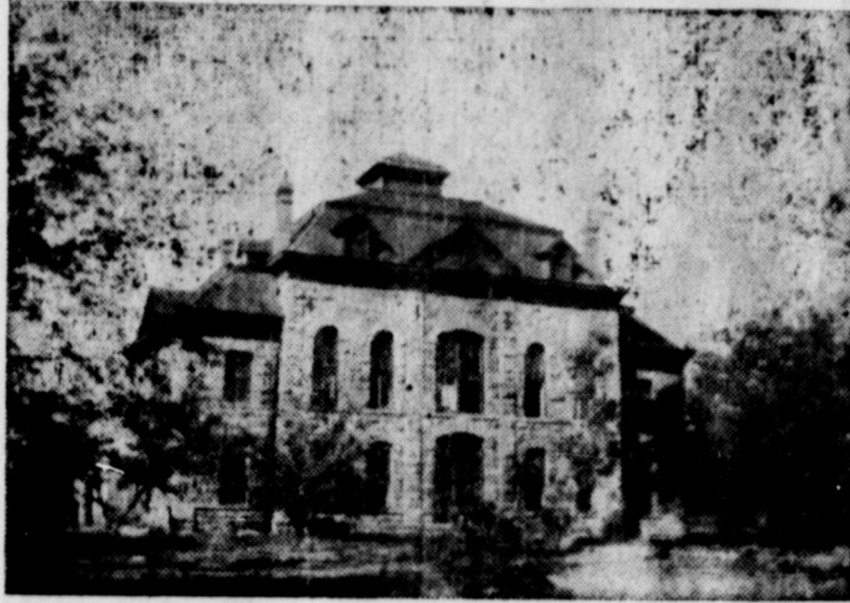
The Coke County courthouse at Robert Lee is built of native stone and is sufficient in size to care for the various county departments, courts, etc.
