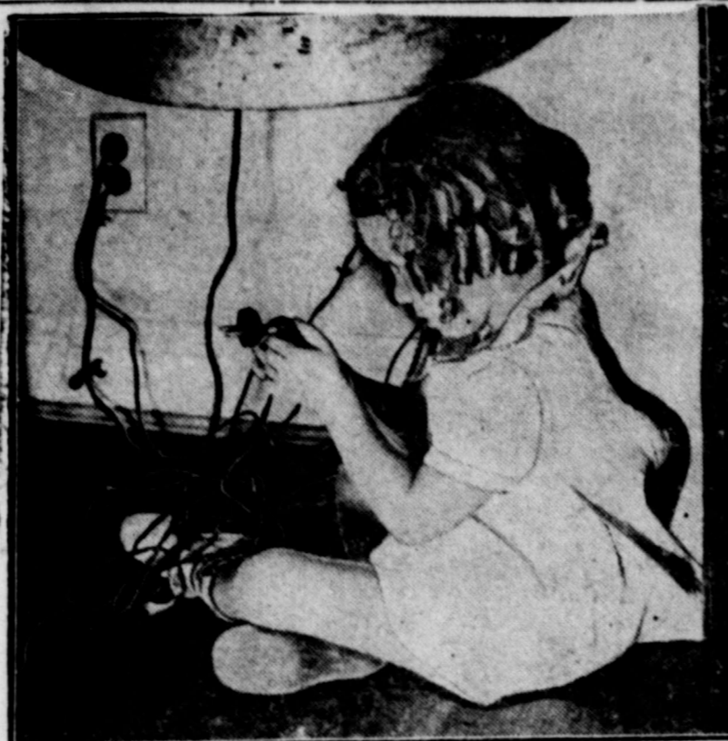
IS YOUR HOME SAFE? —Statistics show that home accidents claimed more lives in 1936 than motor vehicles. Red Cross Accident Prevention campaign is aimed at reducing home hazards. These unprotected and frayed light cords may trip the child or may be short circuited and give her a shock. Red Cross urges all such hazards be checked for home safety.
