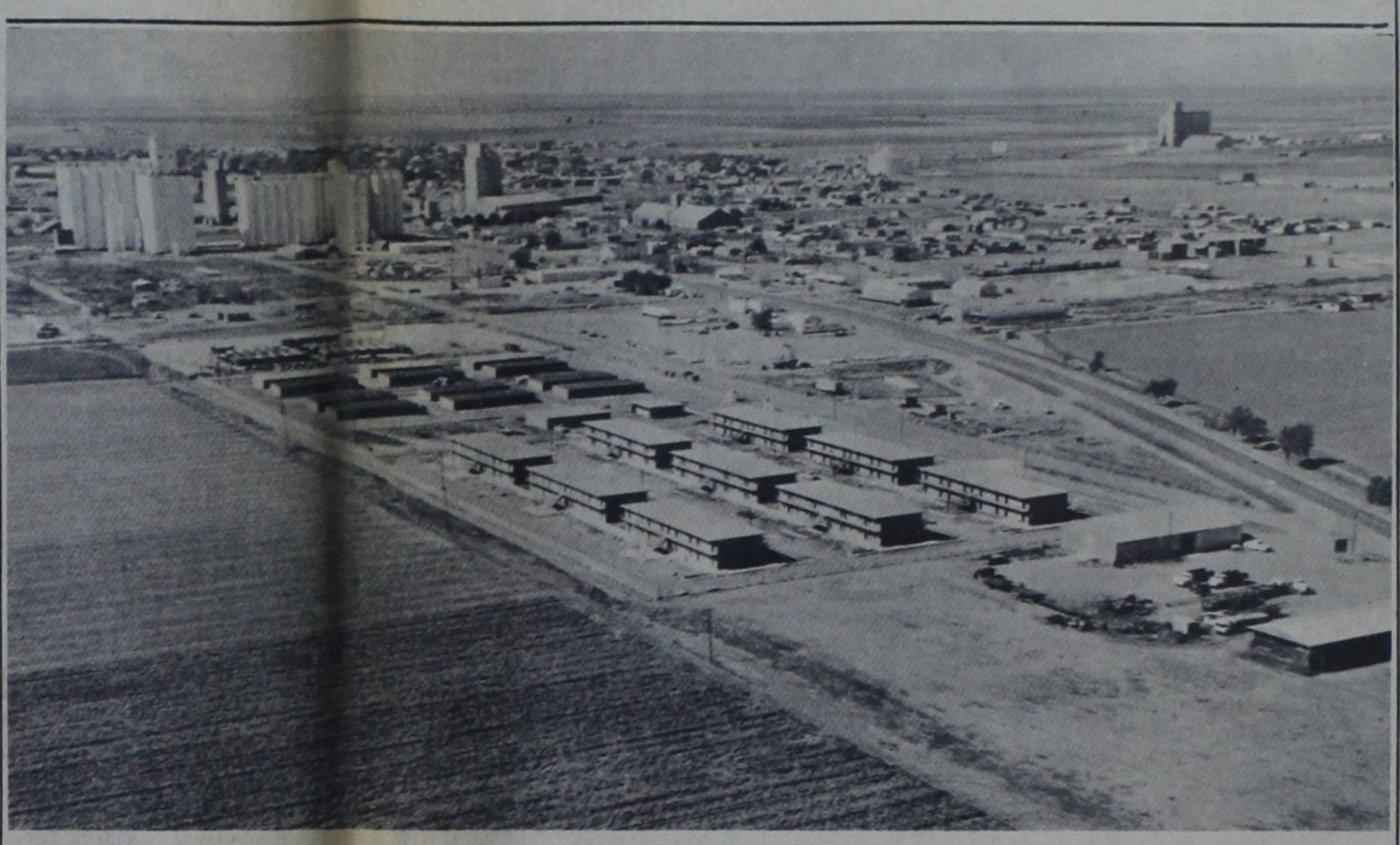
TAKING FINAL SHAPE in East Dimmitt is the huge Castro County Migrant Housing complex, where all 23 buildings are now "off the ground" and ready for finish work. This aerial photo from a Tidwell Spraying Service plane shows the new community within the city much as it will look when completed. The ambitious project, first and largest of its type in the US, consists of nine two-story apartment houses for migrant workers, 12 single-story units for permanent farm laborers, a manager's home and maintenance shop. The county migrant health office will also be located in the $967,000 complex.
