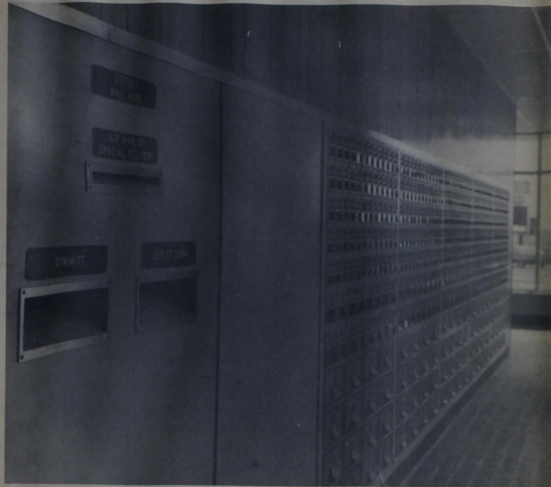
THE NEW POST OFFICE in Dimmitt is virtually completed. Only four light fixtures remain to be installed. This is the
