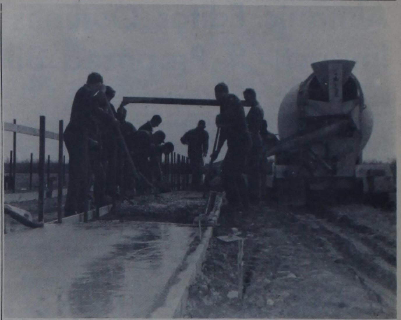
NEW FEEDER PENS for lambs, hogs and calves are being built south of the city limits by Dimmitt High School's FFA boys. Here, an all-day work crew smooths concrete Friday for the walks of the hog and lamb feeder shed, which will have 40 pens to accommodate up to 120 project animals for vocational agriculture students
