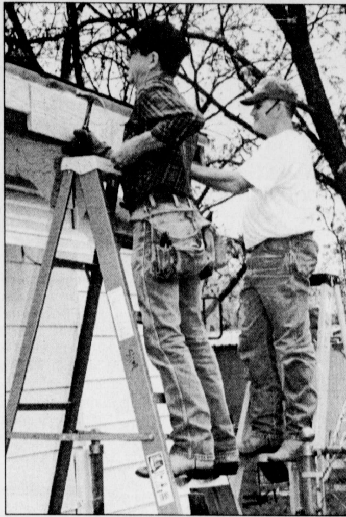
RAYMOND LINDSEY (left) and House Captain Lewis Bergman replace trim around their CIA home.
