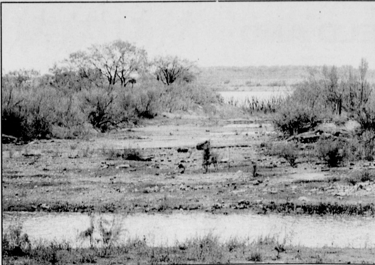
NICE BUT NOT QUITE ENOUGH — YET is the look of the spillway from the old Winters Lake which flows into Elm Creek Reservoir (in background). Despite recent rainfall and days of drizzle, the lakes have failed to catch enough rain to significantly raise the water levels.
