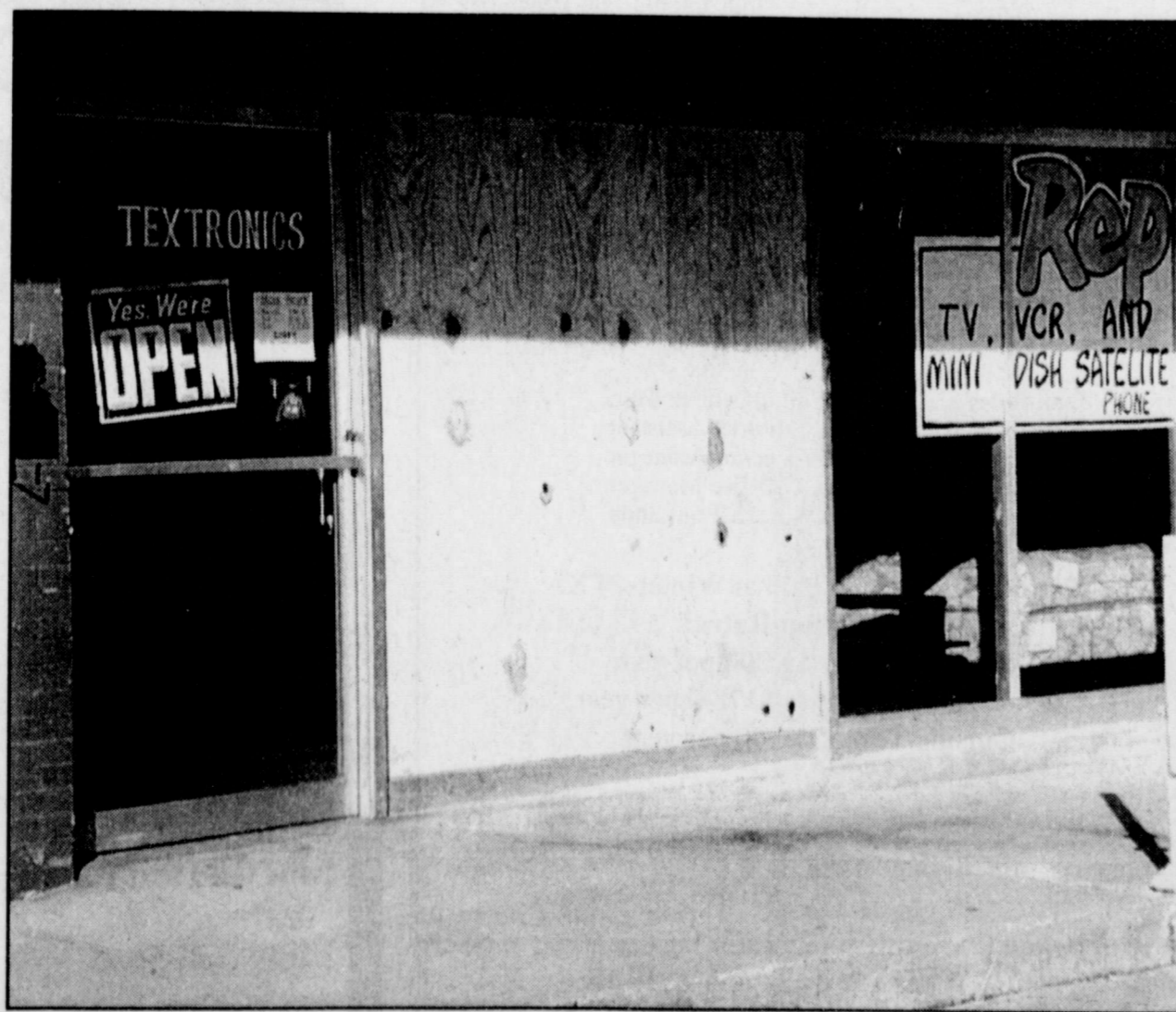
TEXTRONICS, located at 120 West Dale, uses plywood sheets to temporarily replace a large plate glass window broken during a rampage of burglaries discovered early Nov. 15. At least four downtown businesses were damaged by the vandals.
