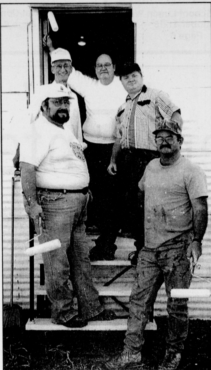
"THE HOLY ROLLERS", as they like to be called, recently painted part of the old Foxworth-Galbraith building on Church street in preparation for the new home of the Winters Food Pantry. Painters and ministers include (clockwise from lower left) Bob Jones of the Assembly of God, Robert Sherman of the Winters Christian Fellowship, Vernon Groce of the Church of God, Don Roath of the First United Methodist Church, and Jim Hanson of St. John's Lutheran Church. The charitable pantry, sponsored by the Winters Ministerial Alliance, will celebrate its grand opening on Monday, Oct. 18.
