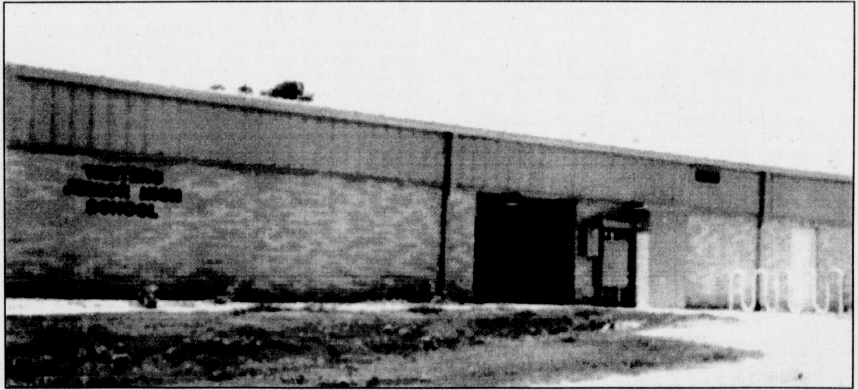
NEW JUNIOR HIGH SCHOOL BUILDING, housing 12,000 square feet, is ready for Winters 7th and 8th grade students to start the new school year on August 12.
