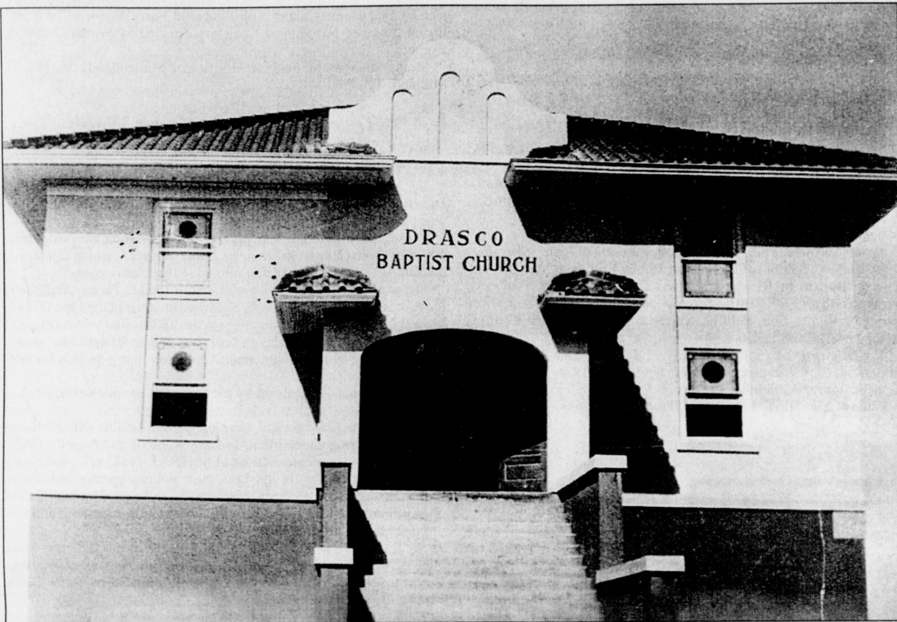
THIS DRASCO BAPTIST CHURCH, built in 1924, was the second church structure for members who first met in the school house in 1907, then moved to a one-room building in 1908. This beautiful two-story church burned in 1951, and was replaced with the present structure which held its final service on May 2, 1999.
