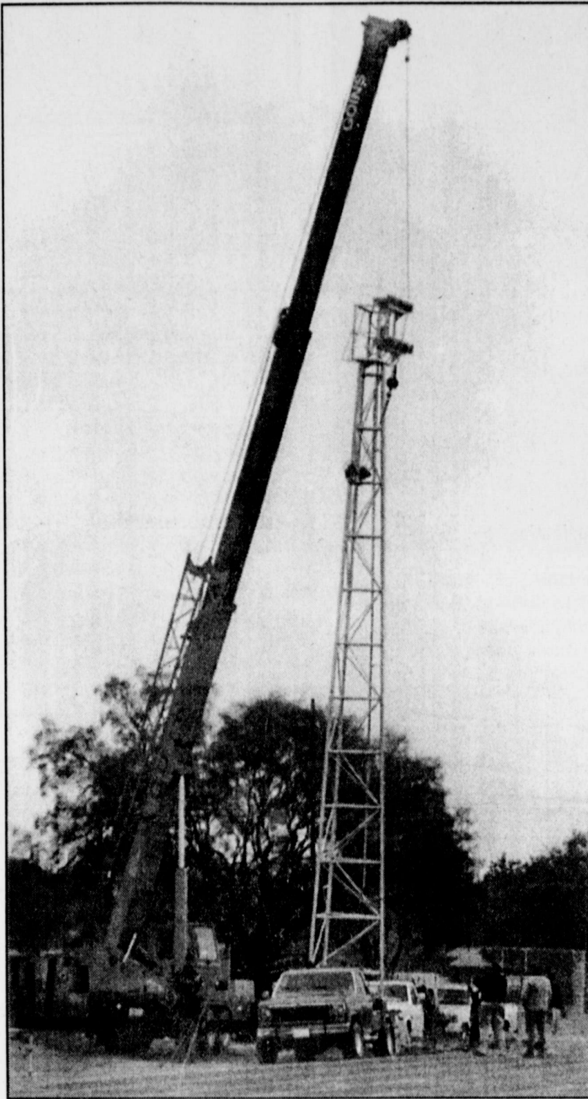
AND LET THERE BE LIGHT! Maintenance crews from WISD work to install the new 55 ft. lighting towers at the Blizzard track field. The four towers house two types of lights —one for recreational walkers and one for official track meet use. The recreational lights will be in operation in about two weeks and will turn on at dusk by automatic timer.
