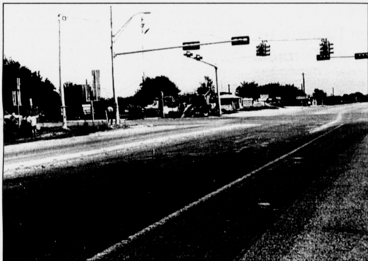
NEW SIGNAL LIGHTS have been installed at the intersection of Highway 83 and 153. The new double signals replace the old fixtures in hopes of improving safety at the busy thoroughfare, and include cameras to monitor traffic in all four directions.
