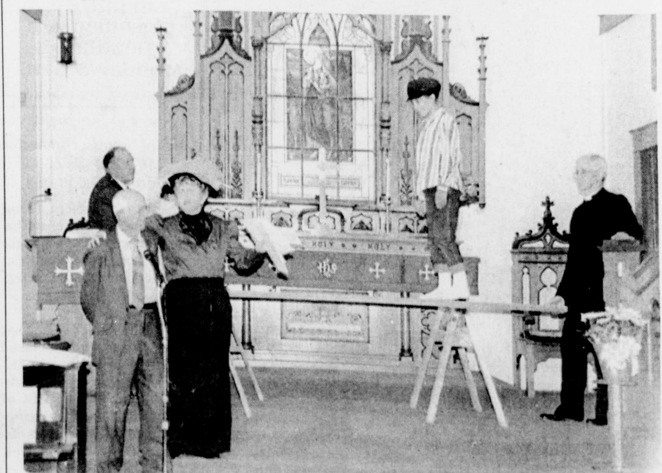
ELLIS UECKERT (standing left foreground) reminisces with Frances Bredemeyer as Heather Watkins reenacts Mr. Ueckert's "walking the center beam" of the church ceiling that was constructed in 1929 when Mr. Ueckert was 19 years old. Mr. Ueckert performed the feat to "prove his daring and agility."
