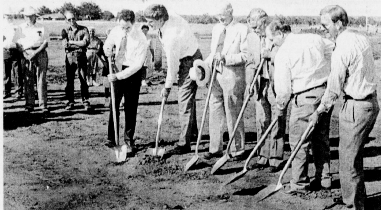
DIGNITARIES GATHERED in Bronte on Monday, August 18 to officially break ground to begin construction of the new Coke County Juvenile Detention Center. Pictured left to right: Wayne Calabrese, Executive Vice-President of Wackenhut; Steve Robinson, Executive Director, Texas Youth Commission; Coke County Judge Royce Lee; State Senator Bill Sims; Gary Compton, Chairman, Texas Youth Commission Board.
