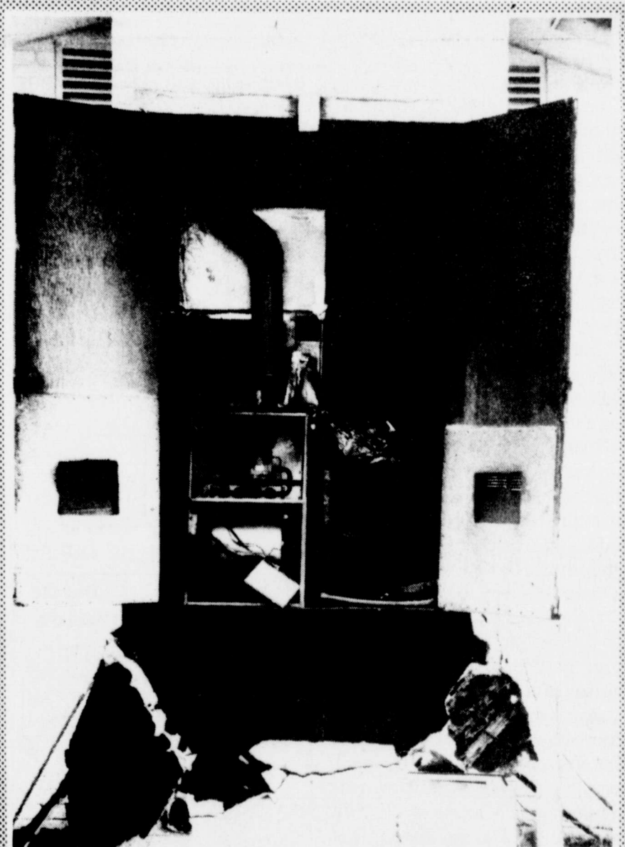
FIRE DESTROYED this large heating unit at the Winters Family Clinic last week. The interior of Dr. Biddix's clinic received smoke damage but no injuries were reported.
