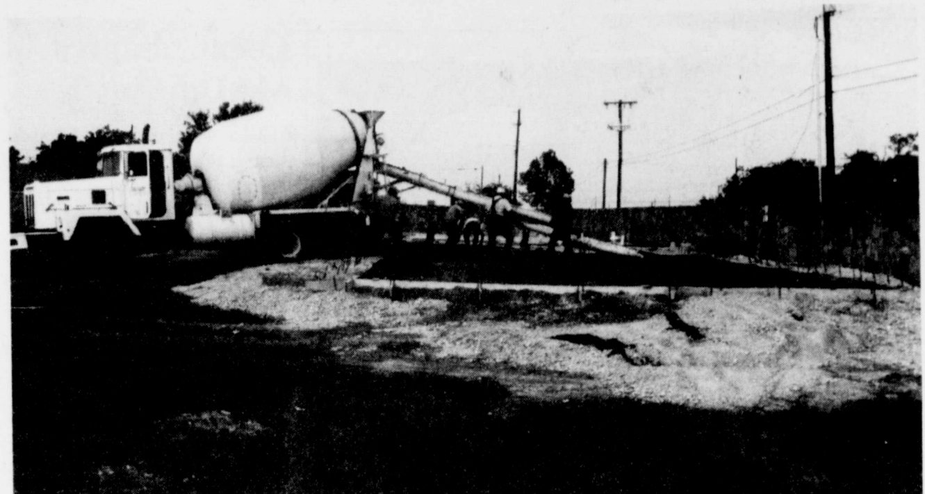
IT WON'T BE LONG NOW—Workers pour cement for the foundation of the new field house at Blizzard Stadium. The building is ready to be delivered and bids are currently being taken for the erection of steel framework. WISD Business Manager Jim Butler has indicated that all work is proceeding on schedule and the finished product will be available for use in the near future.
