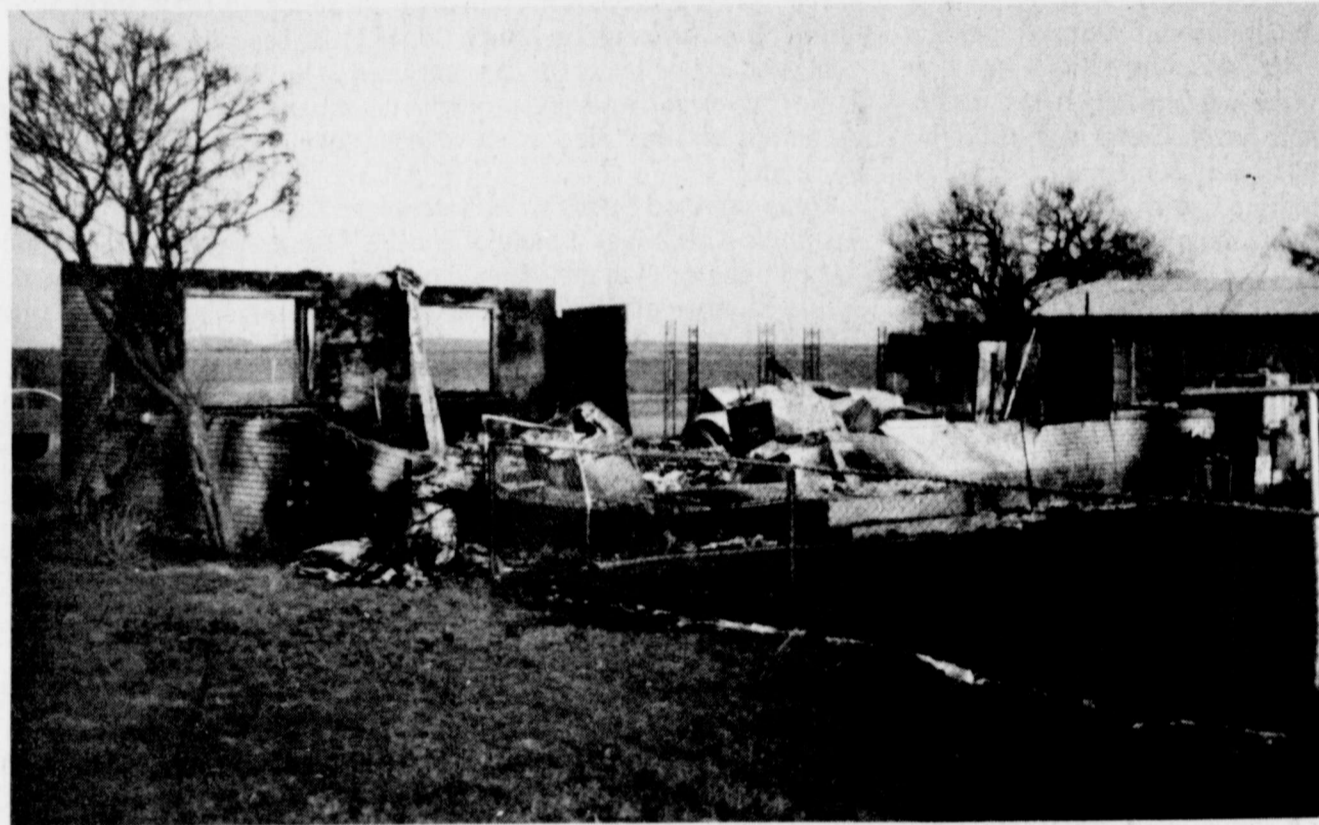
SUNDAY MORNING FIRE — The home of M.F. and Louise Green, located on FM Road 2647, burned Sunday morning while the couple was out of town. Deer hunters called the fire report in at approximately 6 a.m. to the Winters Volunteer Fire Department, but by the time they arrived on the scene, the roof of the house had caved in and the fire was out of control. The property was a total loss and the fire is still under investigation as to the cause.
