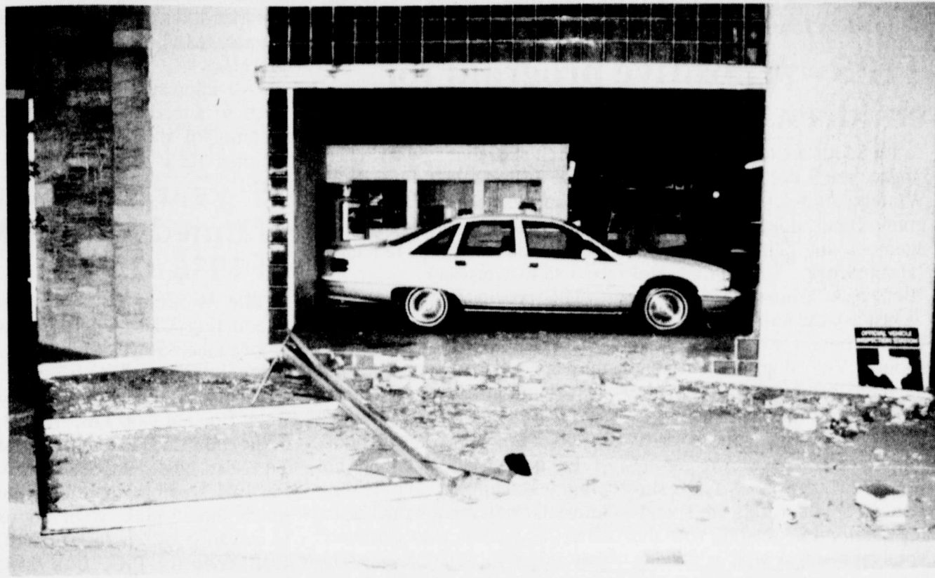
Drive away in a new car? The Charles Bahlman Chevrolet building suffered extensive damage early last Saturday morning when a 17-year old female allegedly burglarized the building, then stole a 1991 Cavalier by driving it through the front plate glass window. See related story.
