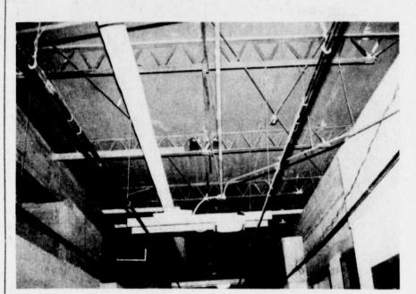
Pictures taken at Winters Elementary School show the apparent deficiencies such as the above where asbestos containing ceiling material was removed, leaving no ceiling.
