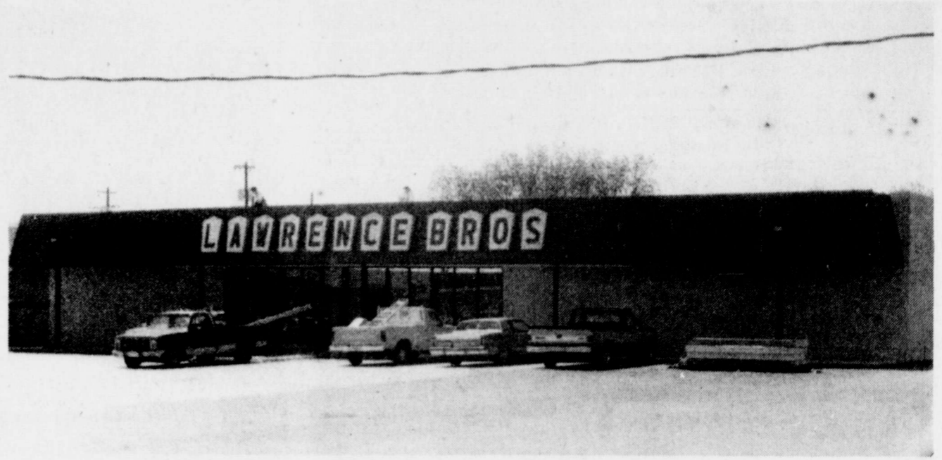
Lawrence Brothers nearing completion.
