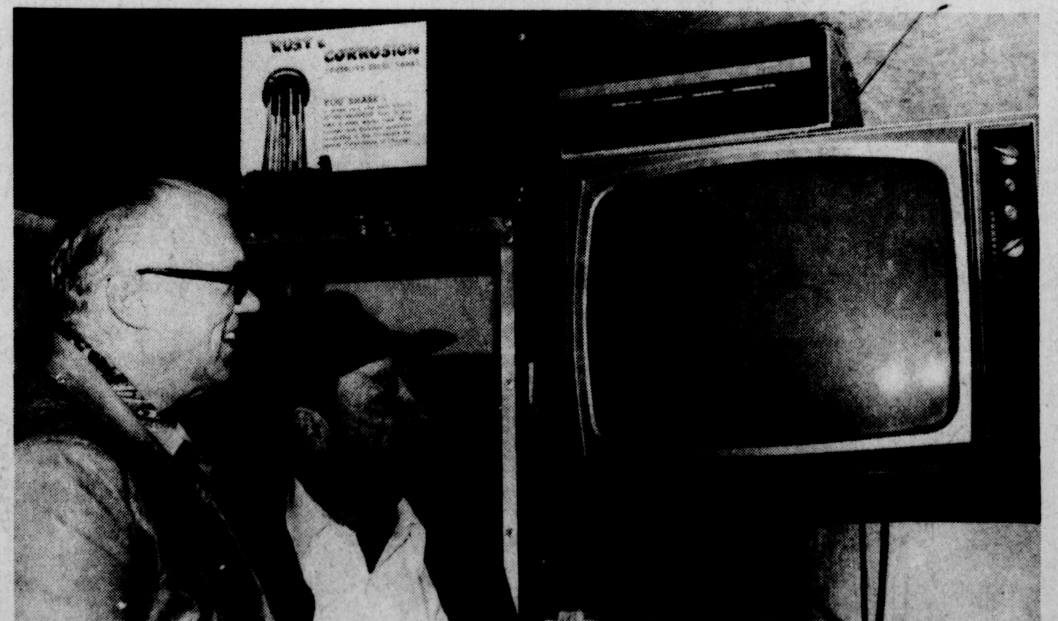
NO. 1 SHOW—Winters Mayor Homer Hodge, left, and Alderman E. J. Bishop watch the closed-circuit television screen as workmen shoot pictures of the inside of the city's south water storage tank. The
