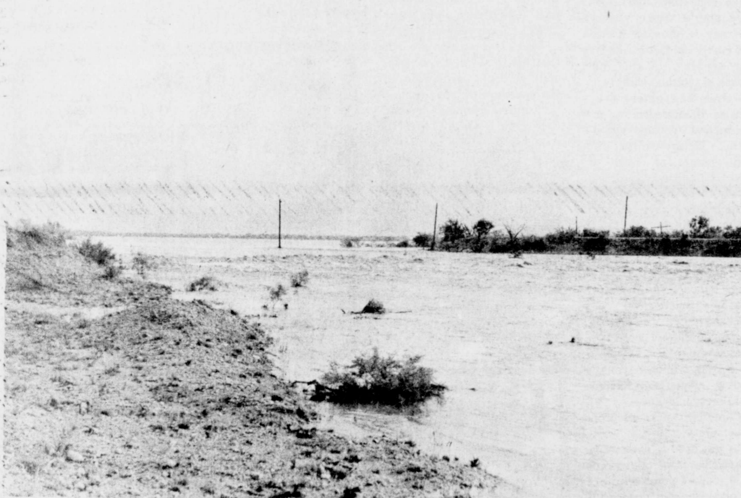
FULL SPILLWAY —The emergency spillway at Winters Lake was filled bank to bank last Friday, following heavy rains. The regular concrete spillway is some place in the middle of this river of water, completely covered.
