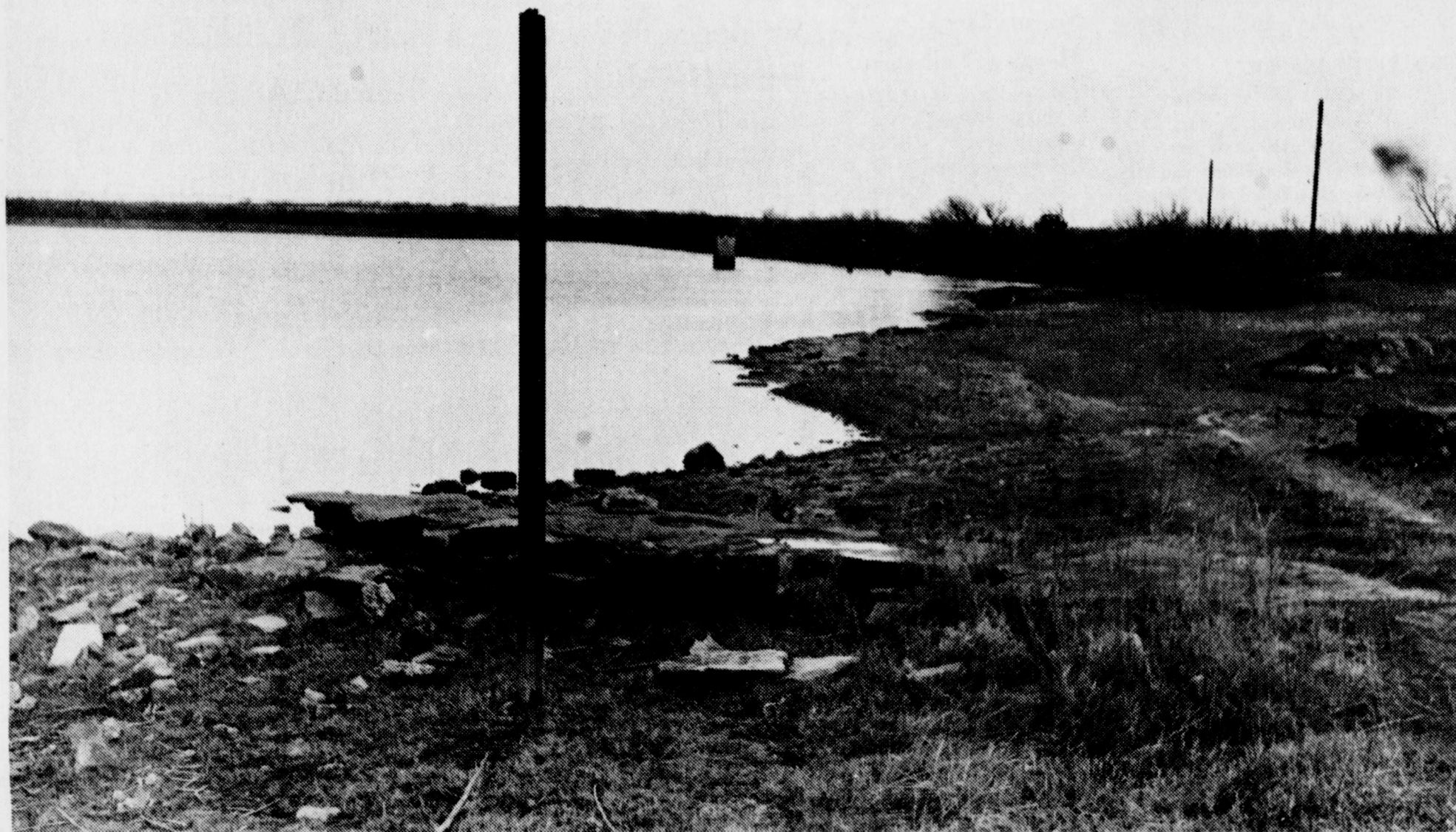
LOW WATER —This picture of Lake Winters, taken a few days ago, graphically illustrates the need for additional water sources. Level of the water is far below spillway level, and with siltation, there is not as much
