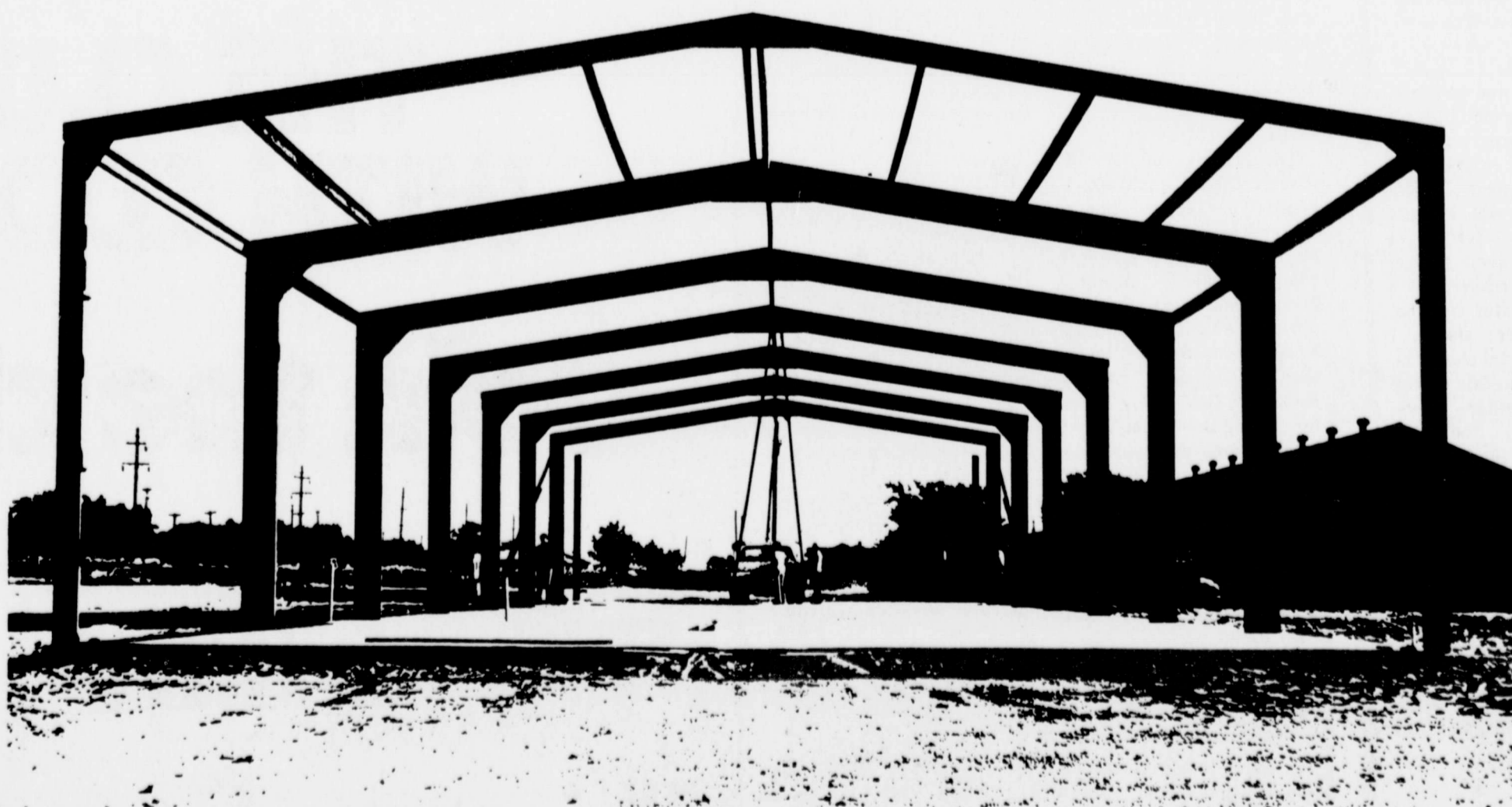
RIBS—Appearing as ribs of some giant animal against the clear sky are the steel girders of the school bus
