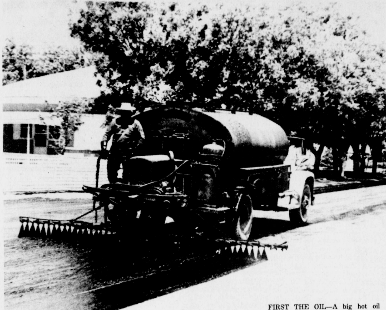
FIRST THE OIL—A big hot oil truck sprays oil on prepared streets to be seal coated . . .
