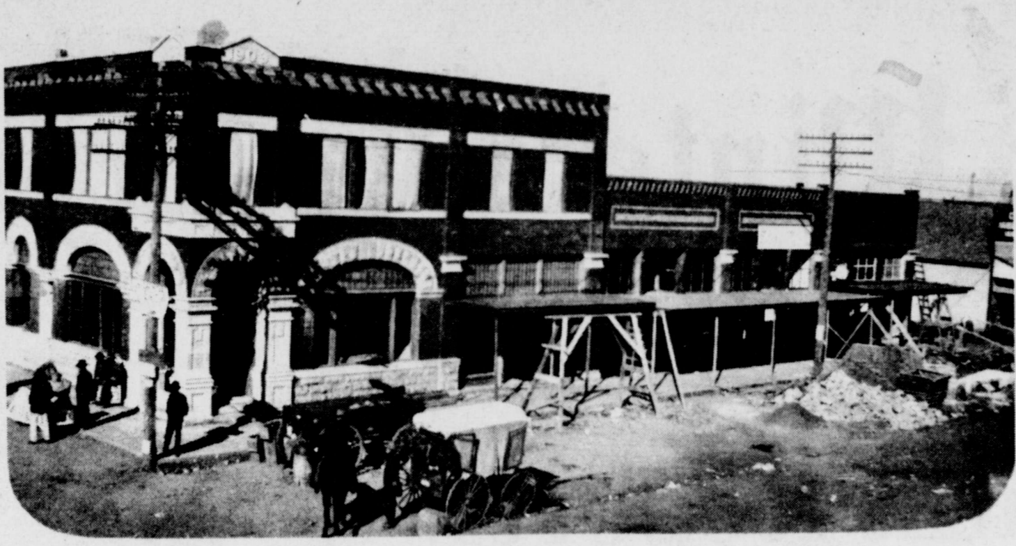
EARLY DAYS —This is a scene of construction of the building housing The Winters State Bank, in 1909. There were no other buildings west of this corner and the railroad, according to the information on the back of the picture. —Photo courtesy of Mrs. Robert Briley.
