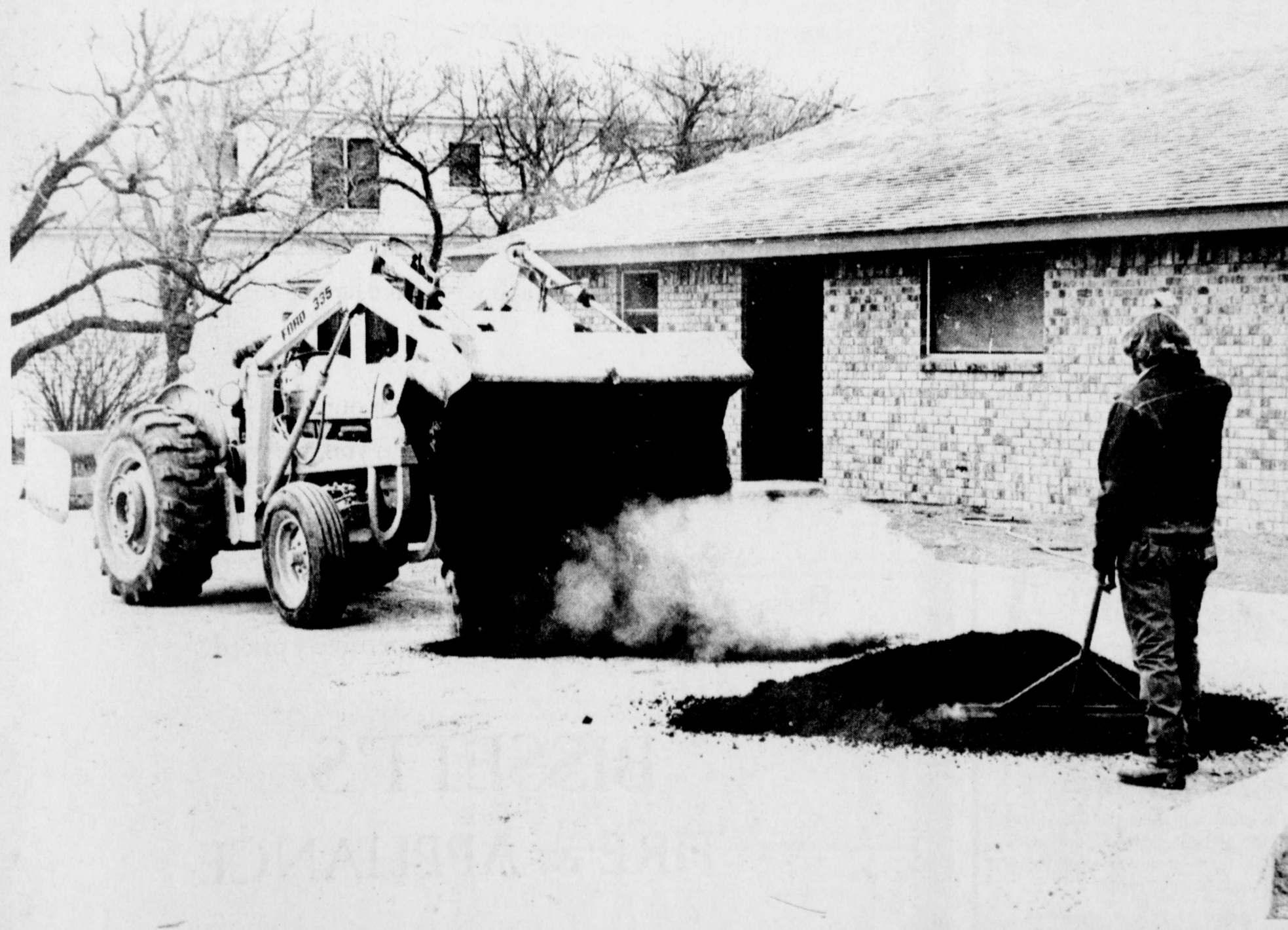
SCHOOL PAVING —Workmen of Bill Walters Paving Contractors of Coleman distribute
