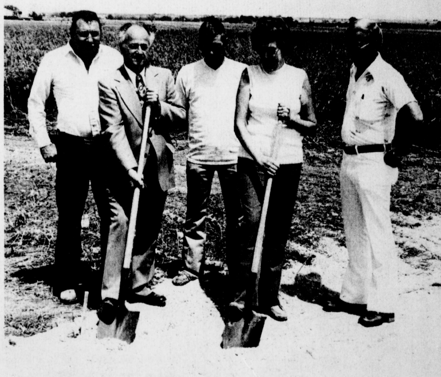
GROUNDBREAKING—Members of the building committee of the Winters VFW post, the president of the VFW Auxiliary, and designer of the new post home, break ground for the new $45,000 building. With shovels are
