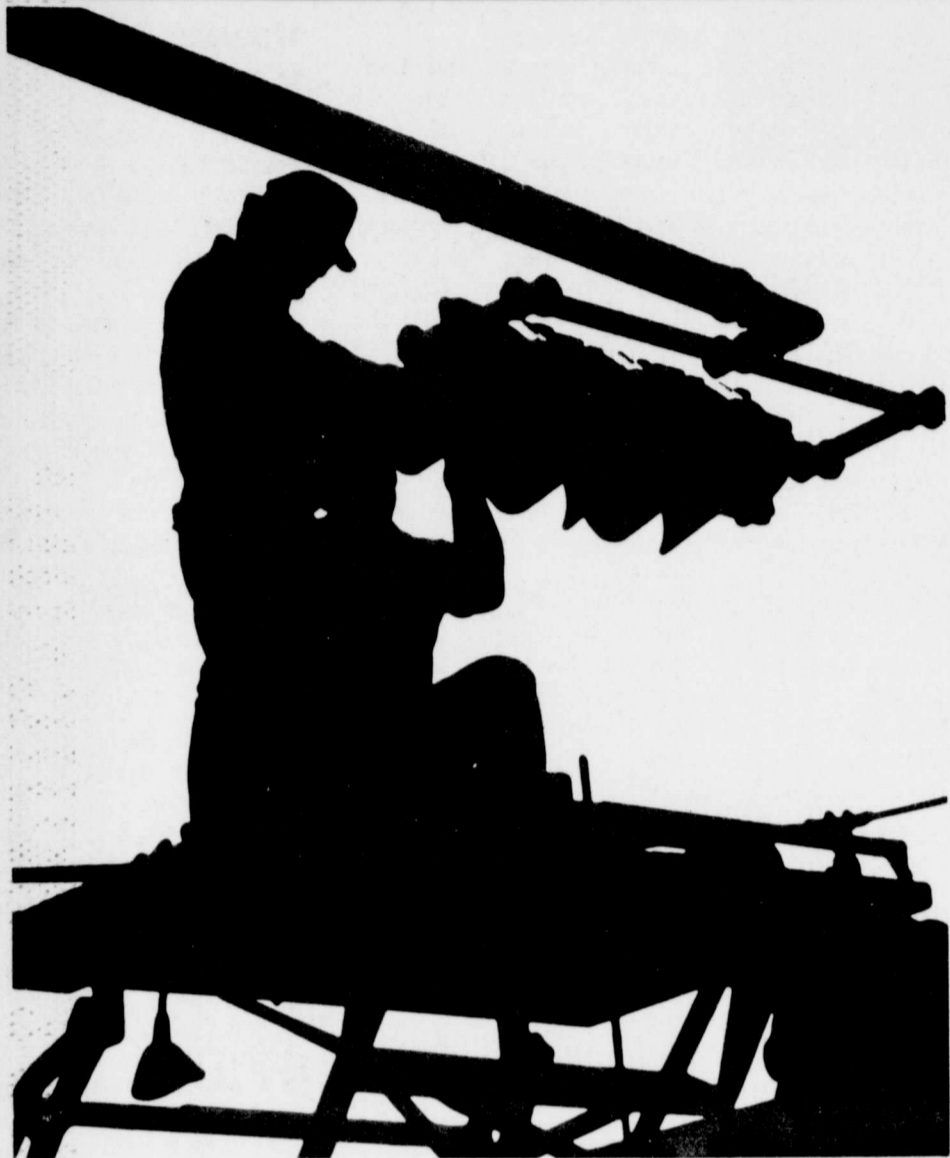
LIGHT WORK —The photographer's silhouette treatment of Highway Dept. workmen installing the new traffic lights at the corner of Main and Dale streets lends strength and depth to what might have been an ordinary
