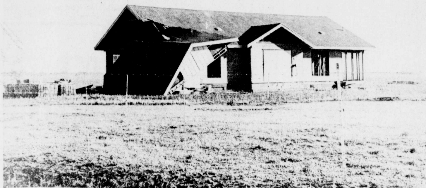
DESTRUCTION OF NEW CONSTRUCTION—A new house under construction by George Brown, across the FM road from the
