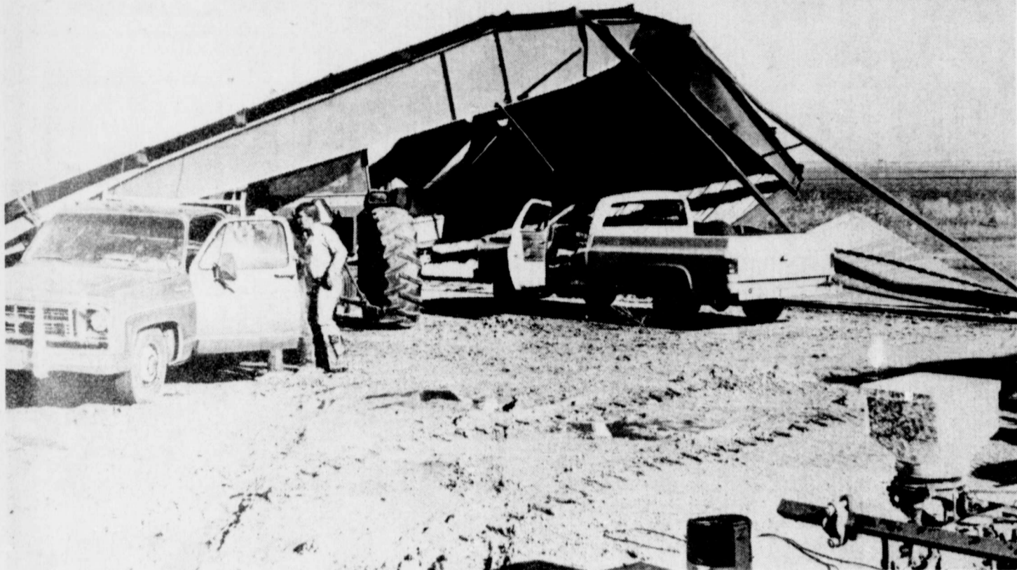
DESTROYED —This is the big metal implement shed on the Raymond Schwartz place north of Winters following the tornado which swept through last Thursday afternoon. The building was completely destroyed; metal girders were twisted like pretzels, and rolling equipment which was in the building was damaged.
