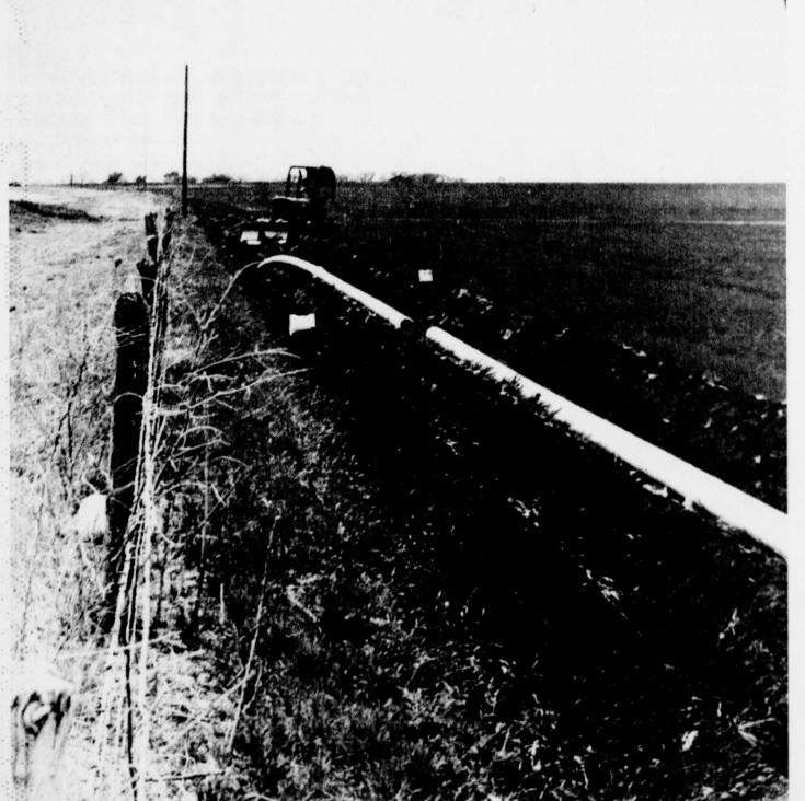
PIPELINE-White pipe which will carry water to rural homes in North Runnels lies ready to be pushed into the ditch and connected, just ahead of the motor blade which will cover the ditch. The picture was taken from just behind the ditch digger, as crews of R. T. Swelling & Sons of Whitney completed the first three days of construction on the
