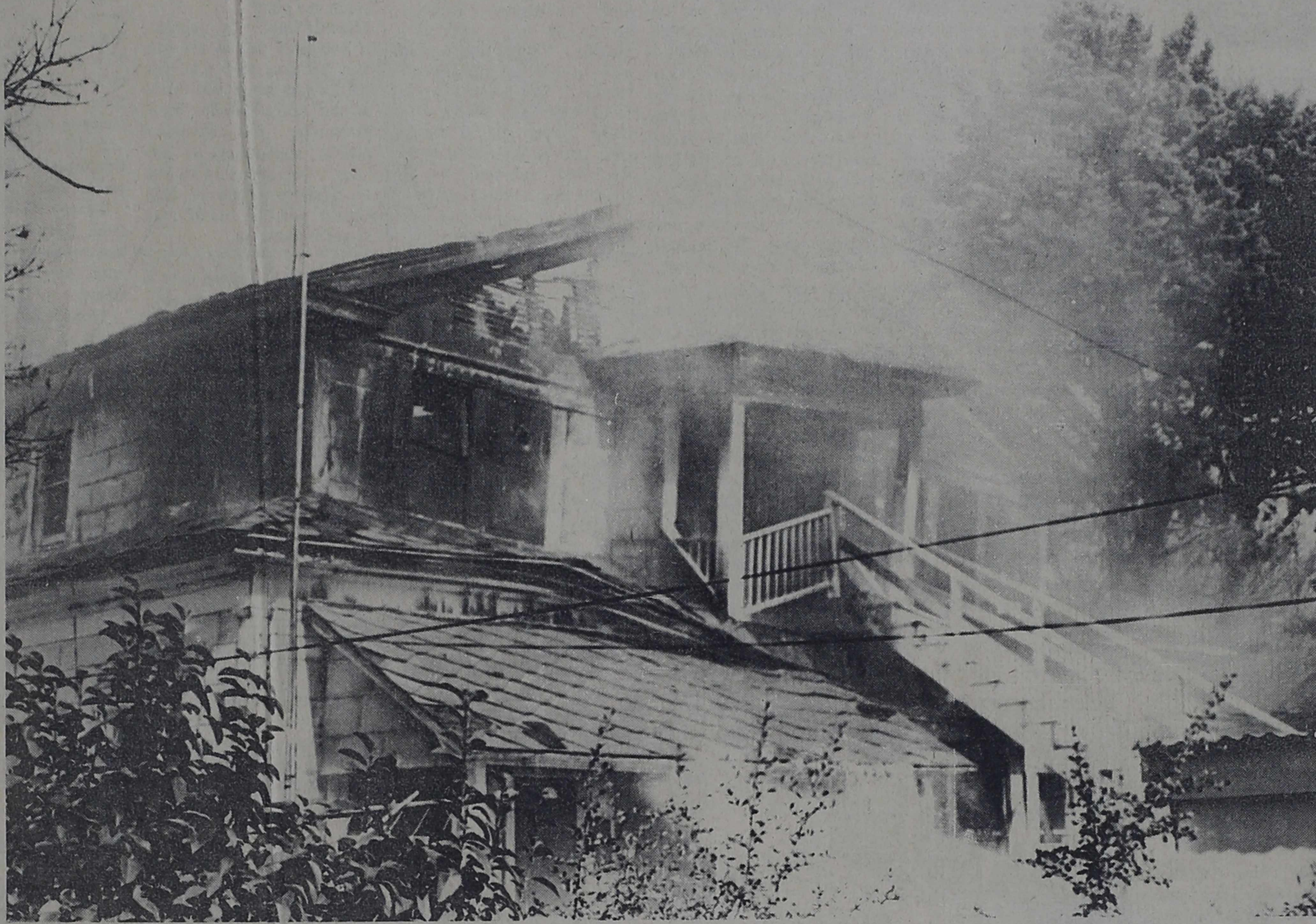
FIRE! —Only outside walls were left partially standing after fire Sunday gutted this two story house on South Arlington. Firemen battled the flames for at least five hours. It has not been
