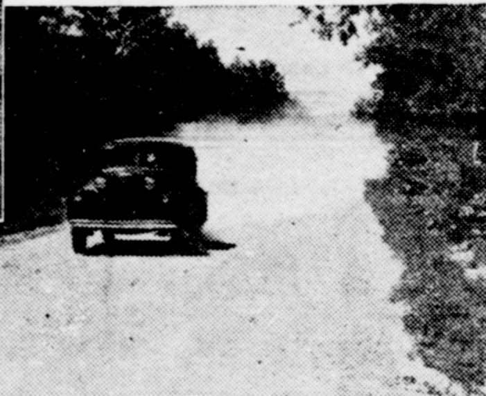
Left—Science has proved that mixtures of natural soil materials, held together by moisture, can convert this typical mud "road" into one that is as dustless in August as it is mudless in April.
