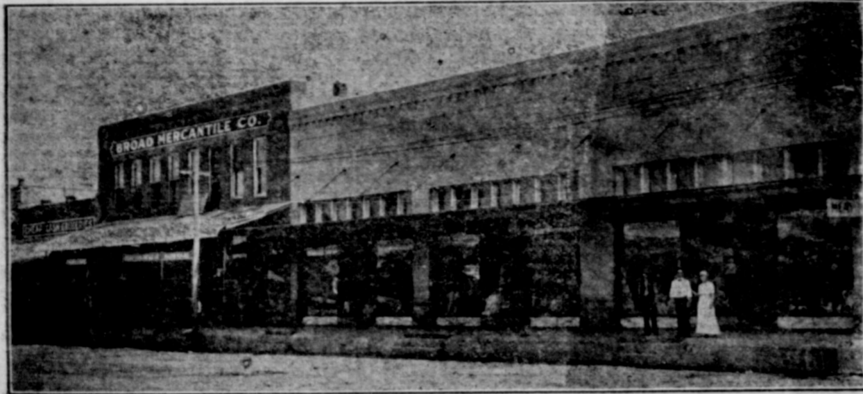
VIEW OF SOUTH SIDE SQUARE BRADY
