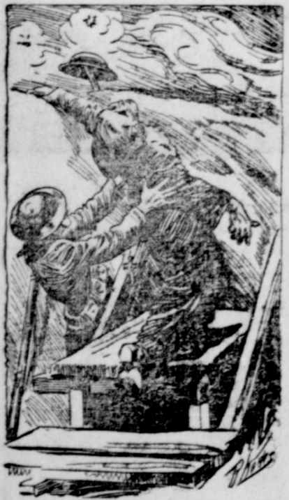
Stuck His Head Over the Parapet and Got It Square.
