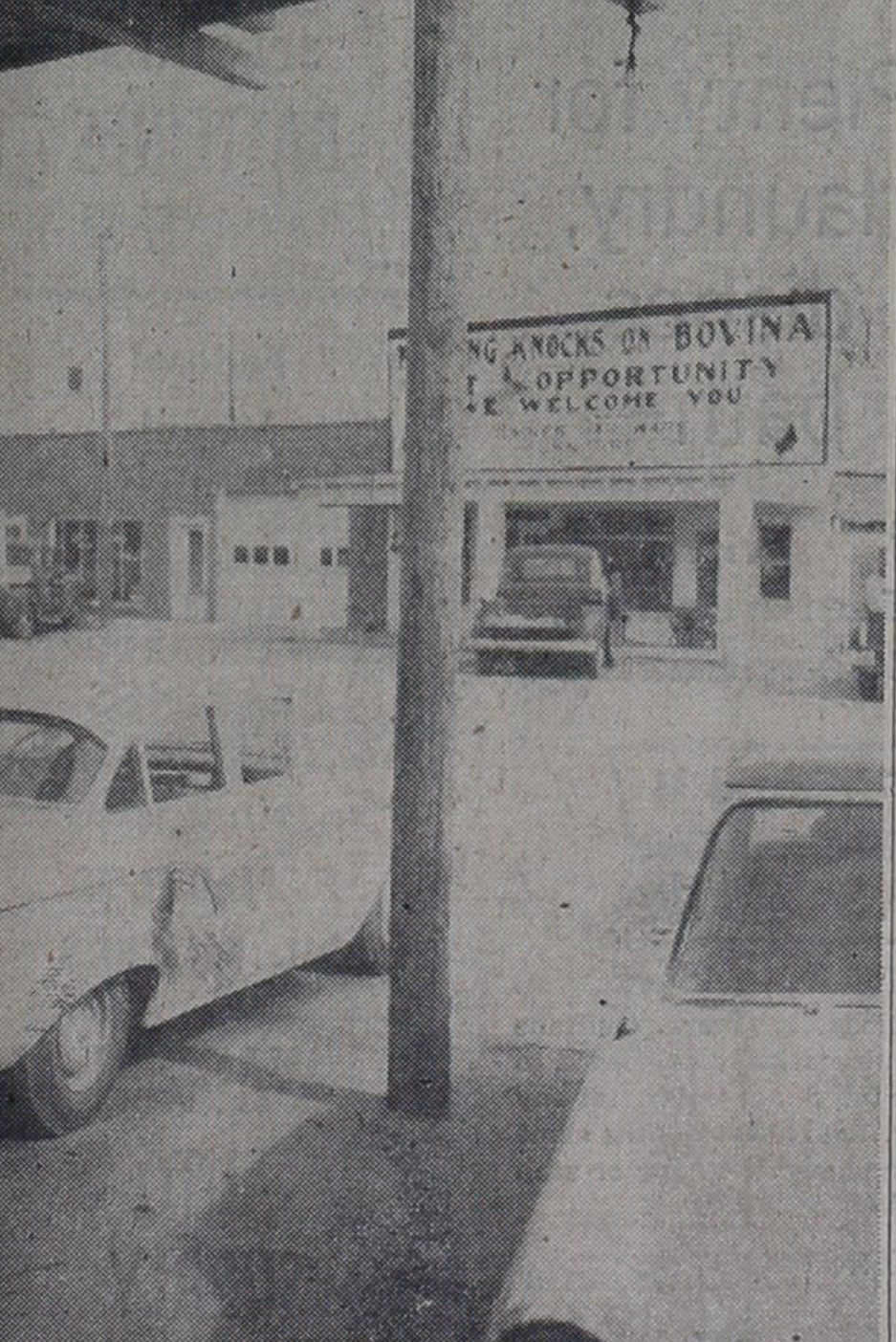
POLES TO BE MOVED—Poles for telephone and power lines are to be moved from the northwest side of Bovina Main Street, and as shown here, more parking space and better looks will be added to the main drag.
